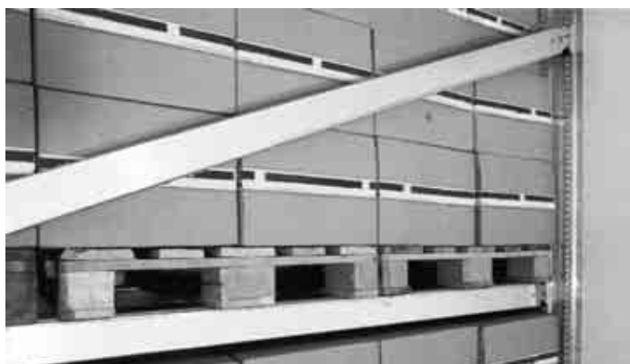
Blocking with liftable loading platform beam.
