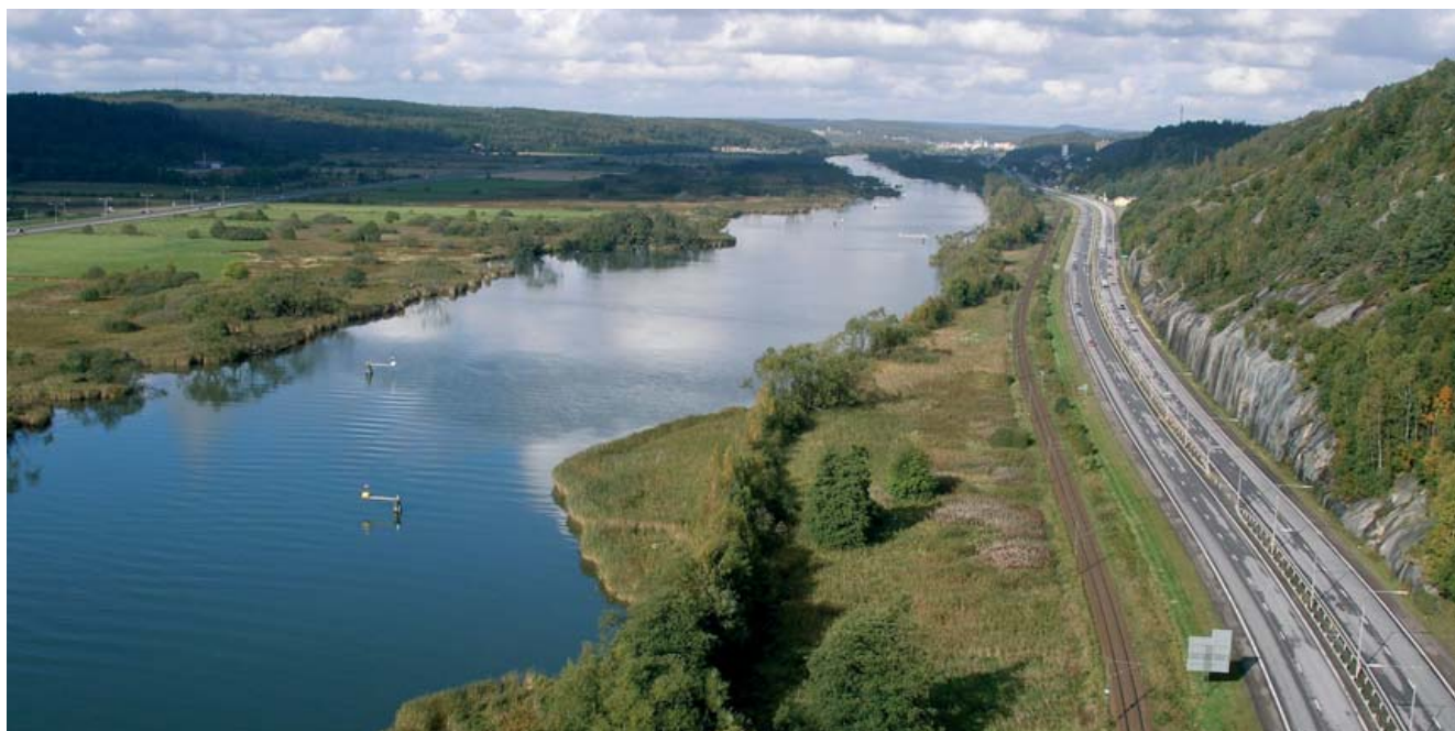
The infrastructure often runs side by side.
