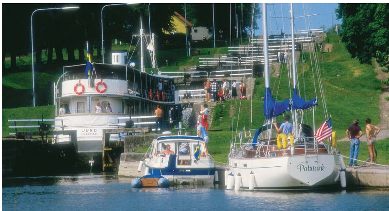
The seven-steps lock at Berg, Göta Canal in Sweden. A picturesque passage for pleasure crafts summertime.
