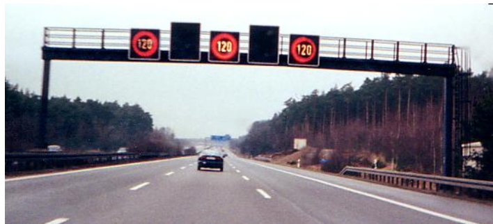
Figure 5-3 : Overhead Speed Control - Germany
