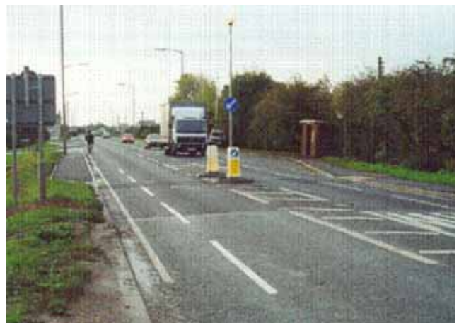
Plate 8 A1174, looking south
