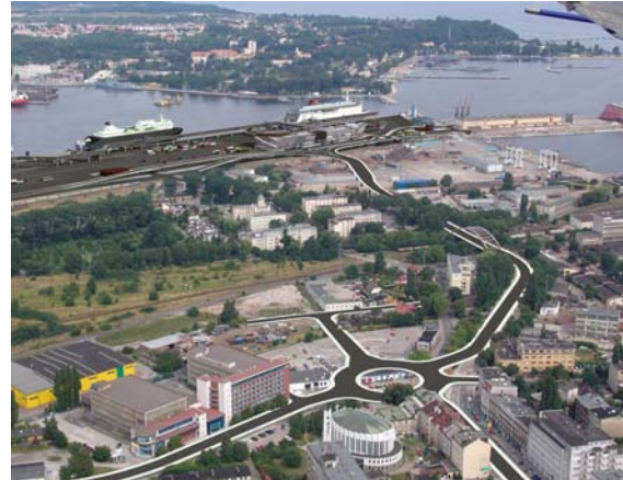
Picture 37: New ferry terminal and road access in the port of Gdynia
