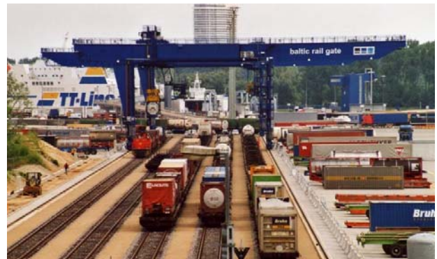
Picture 26: The intermodal terminal in Skandinavienkai, which started to operate in 2003, handles 70.000 intermodal units annually. The capacity is estimated to twice this number.
