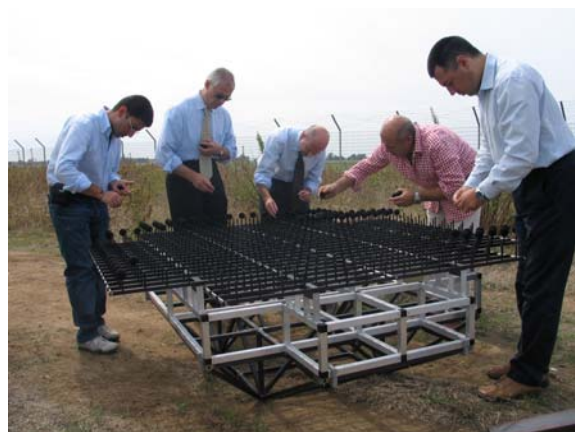
Antenna Assembling On Site
