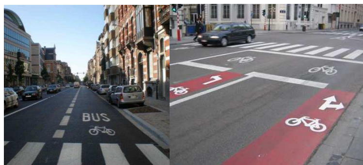
advisory lane, bus/bike lane, advanced stop line – image source: T. Asperges, D. Dufour
