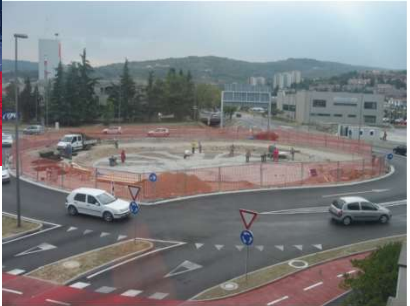
The first Slovenian Turbo Roundabout - under construction; city Koper 2008
