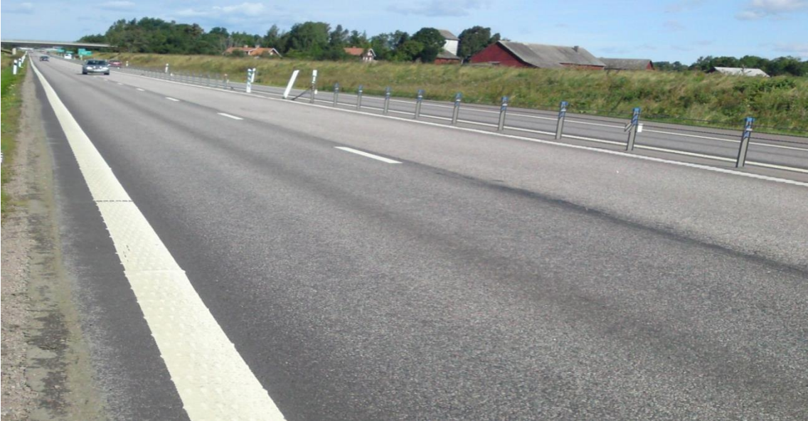
Photograph 4. Ref 1b. (Photo. Terence McGarvey).
