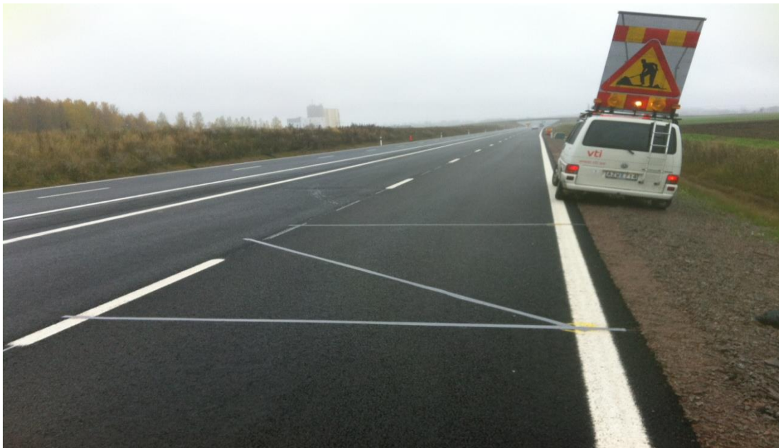
Photograph 13. Ref 6b. (Photo. Terence McGarvey).
