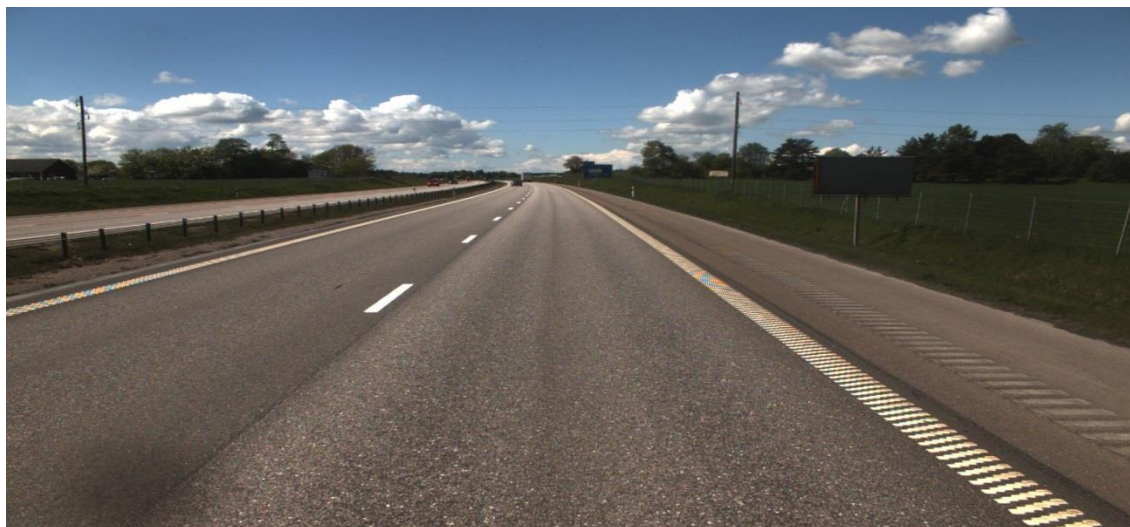
Photograph 11. Ref 5b. (Photo. Trafikverket PMSv3).
