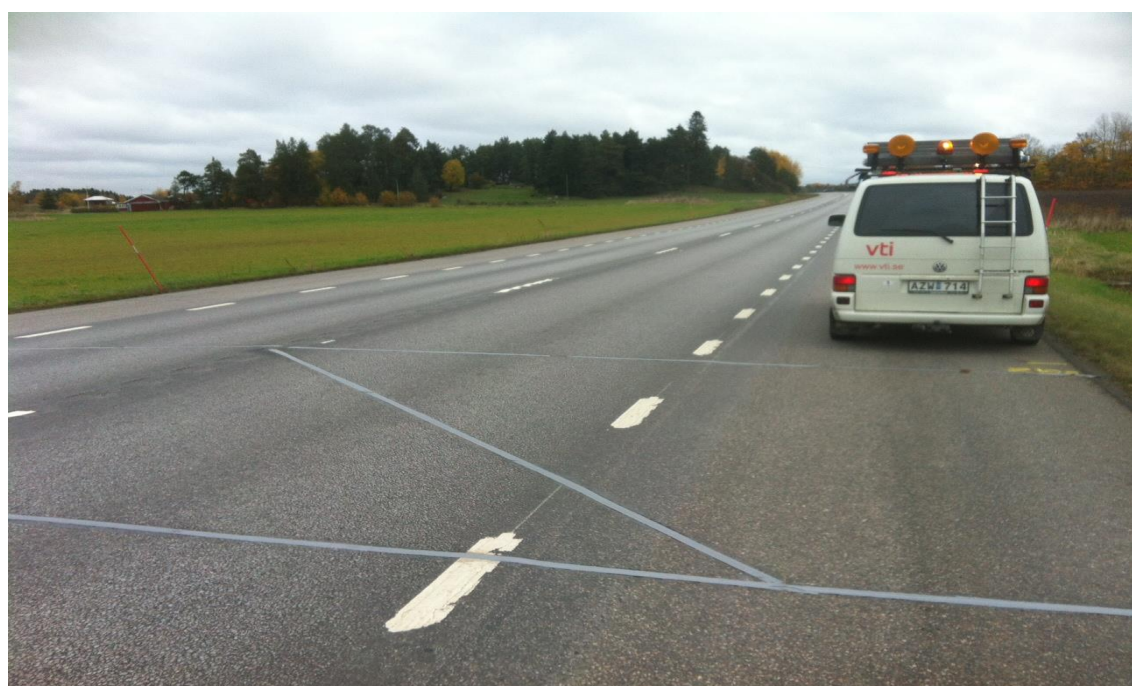
Photograph 14. Ref 7a. (Photo. Terence McGarvey).
