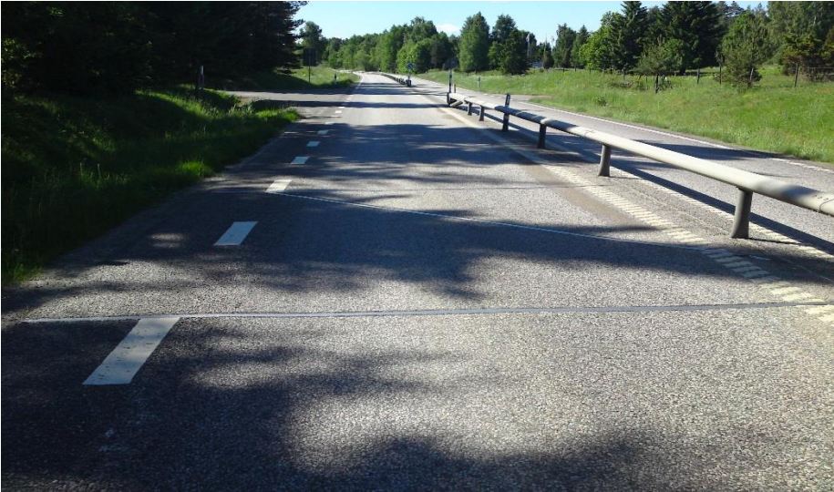
Photograph 8. Ref 3b. (Photo. Terence McGarvey).
