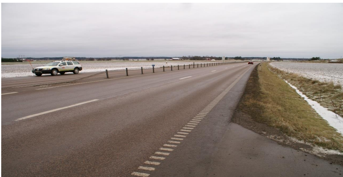
Photograph 6. Ref 2b. (Photo. Terence McGarvey).
