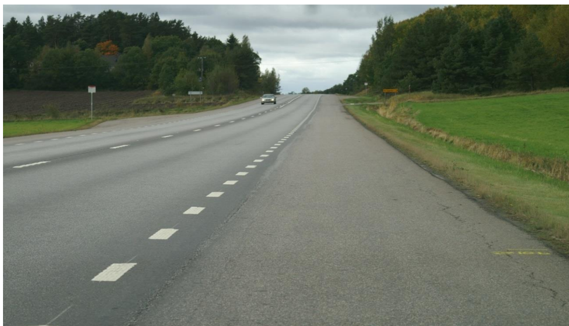
Photograph 15. Ref 7b. (Photo. Terence McGarvey).
