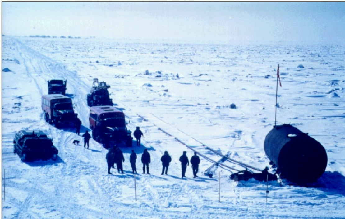
Figure 24 Winter road along the gas condensate pipeline laid over the ice
