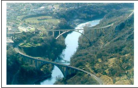
River Soèa Bridges, Slovenia
