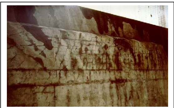
Alkali silica reaction
