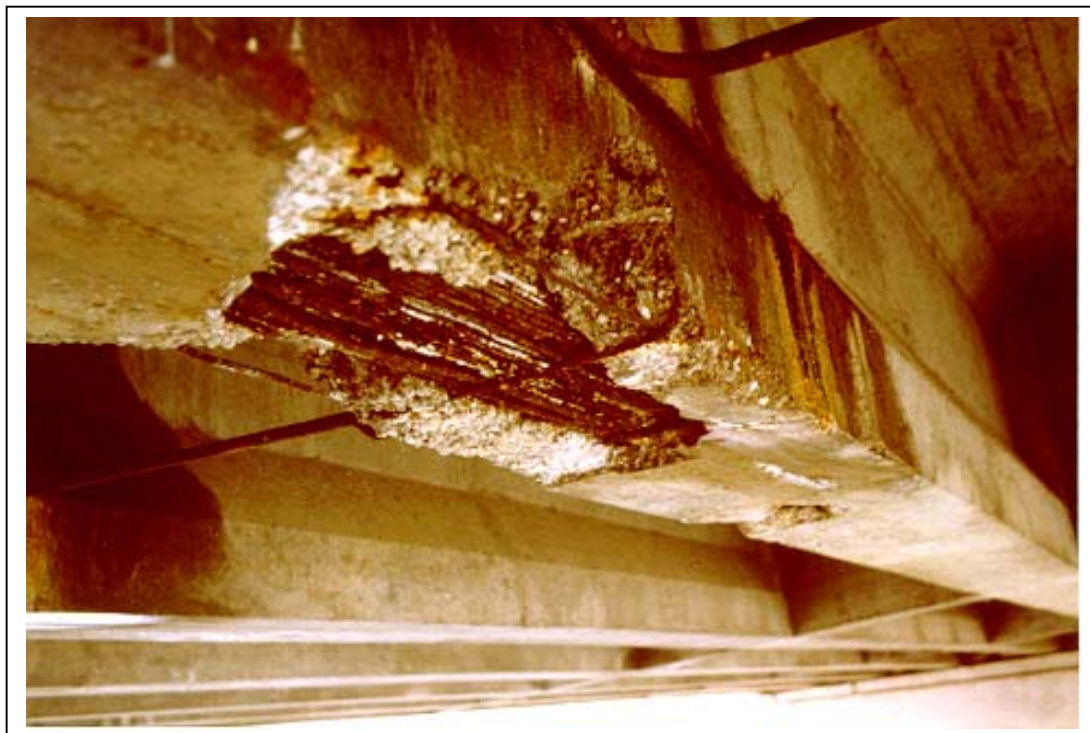
Figure 2.1: Corrosion of a prestressing tendon
