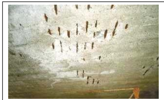
Reinforcement corrosion
