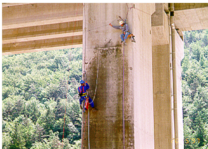
Figure 3.7: In-depth inspection of piers by abseiling
