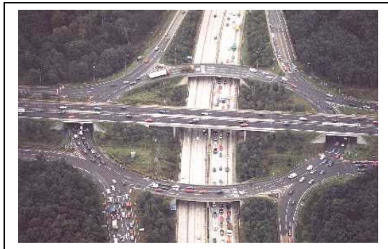
Grade separated junction, UK
