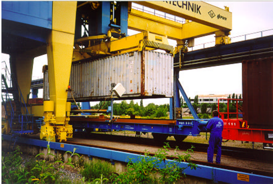
Fig. 4.9.5/3: Wagon 222 in Automated Terminal
