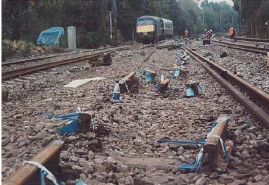
Figure 1: The Hatfield rail track site following the accident [taken from Ref. 1].
