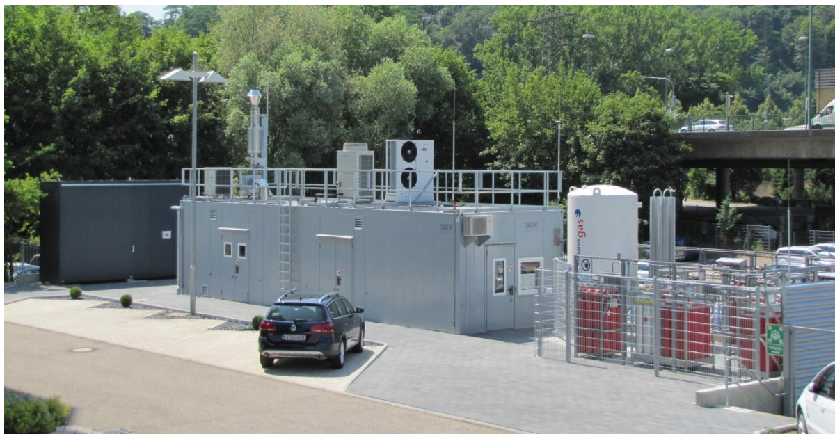
Figure 8: New laboratory for fuel cell systems (Eberspächer)
