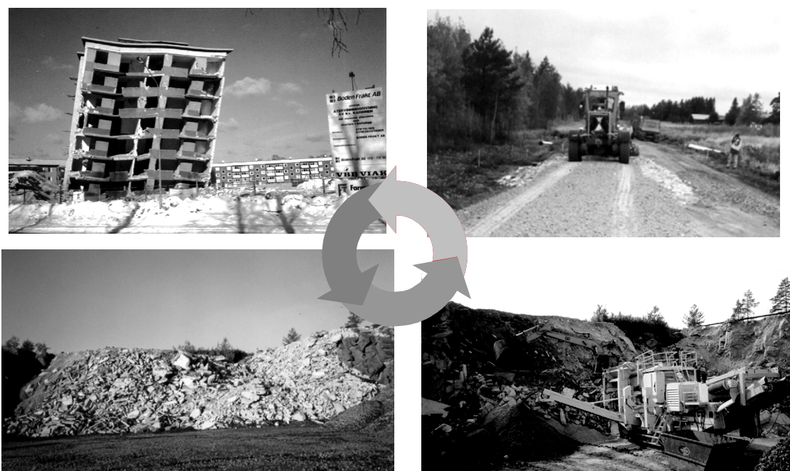
Figure 7.16 Recycling strategy: "The Leaning House of Boden" used as sub-base in test sections
