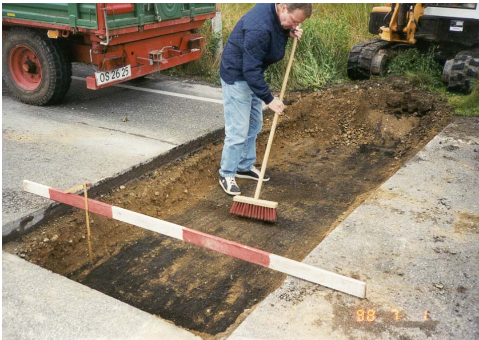
Figure 7.21 Excavation for investigation of existing road, Denmark
