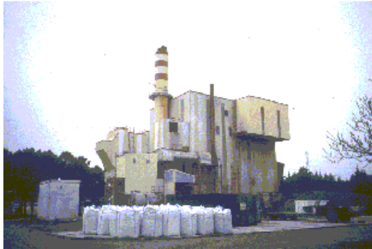
Figure 7.3 La Teste incineration plant and the inspected road
