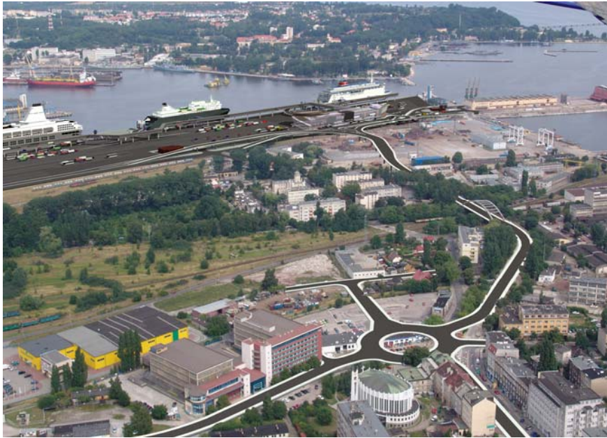
Photo montage of the planned terminal expansion and road connections to the port in Gdynia. The railroad is already of a sufficient standard to handle goods traffic.
