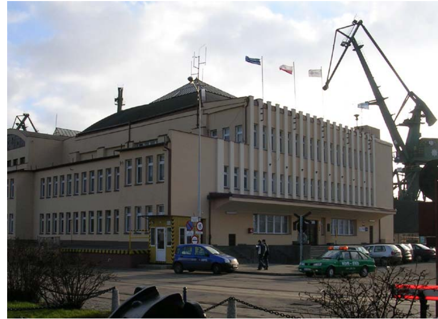
The America terminal in the port of Gdynia
