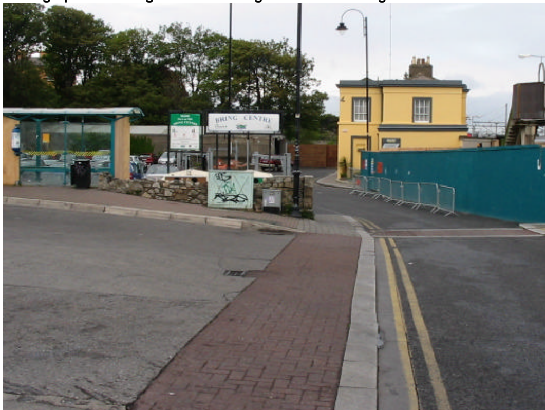
Photograph 1: Existing Station Building and PT Interchange
