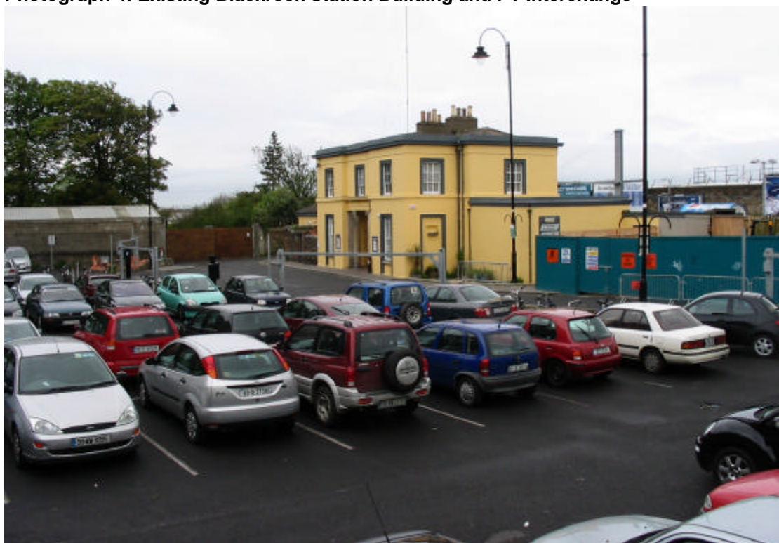
Photograph 4: Existing Blackrock Station Building and PT Interchange
