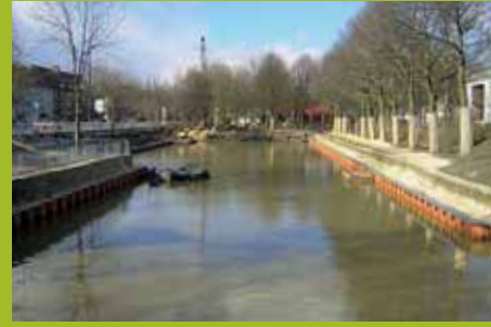
Construction of the Peat Harbour at Findorff
