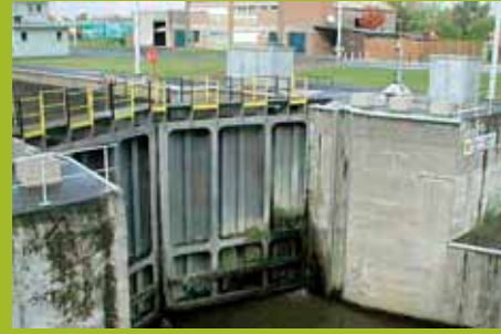
The modern 'Freight' Lock at Ooigem
