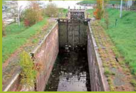
The Three Steps Lock at Ooigem is being restored
