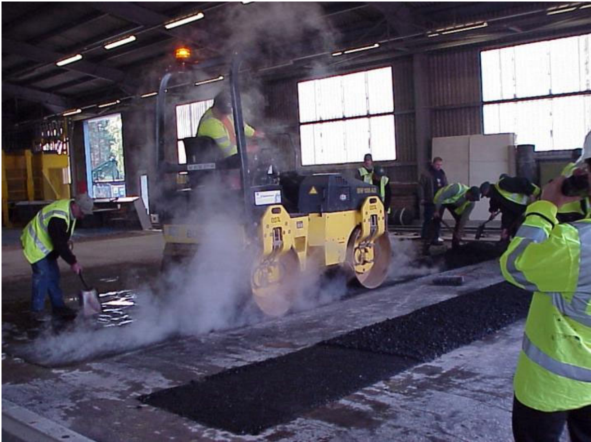
Figure 6.9 - Placing the wheel track HMB15 inlay at TRL
