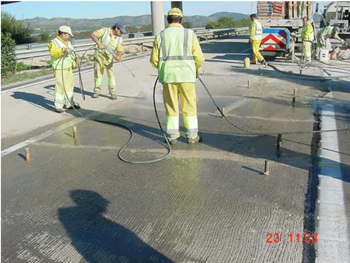
Figure 6.13 – Injection of cement grout
