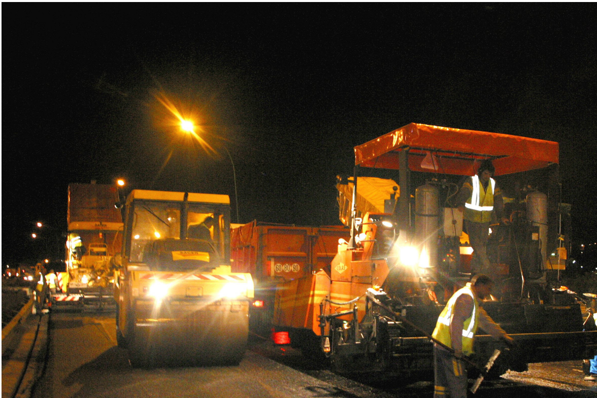
Figure 6.12 – Application of the porous asphalt
