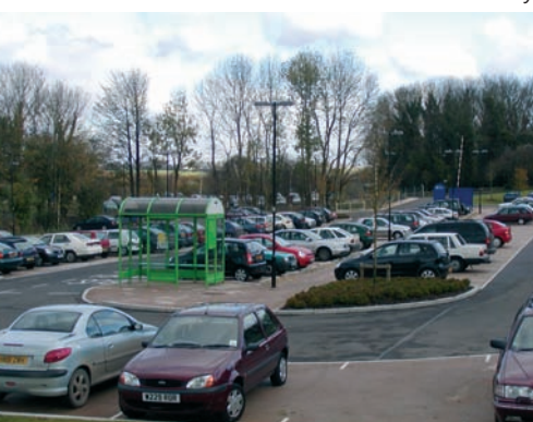
Winchester: "Park and Ride" facility
