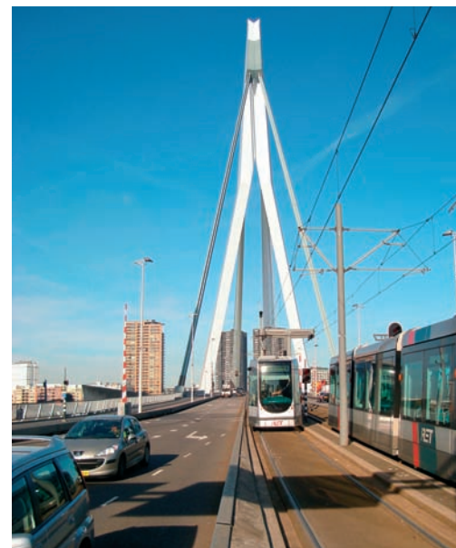
Rotterdam: modern tram lines on the Erasmus bridge
