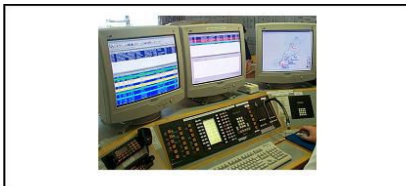
Figure 4 – AIDER integration in Sinelec road control centre
