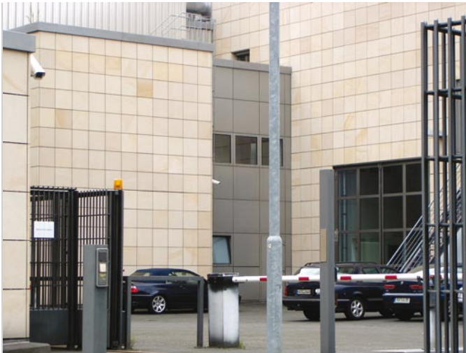
Vehicle access control
