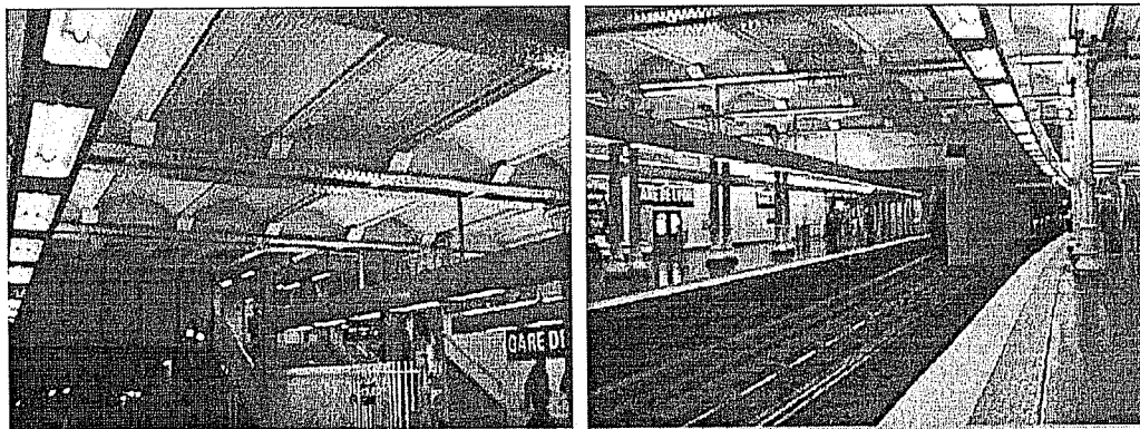
Figure 61 Metallic structures of Gare de Lyon station
