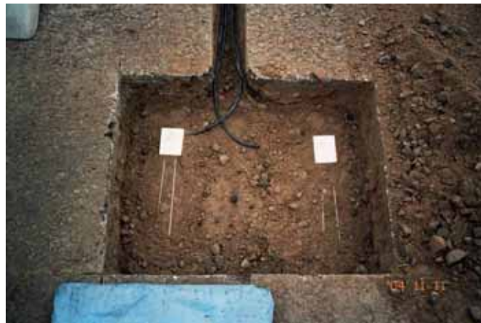
Figure 9: Moisture sensors in unbound pavement at the test site Kindsjön
