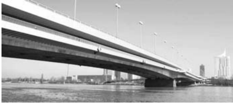
Figure 10: Bridge Reichsbrücke, Vienna
