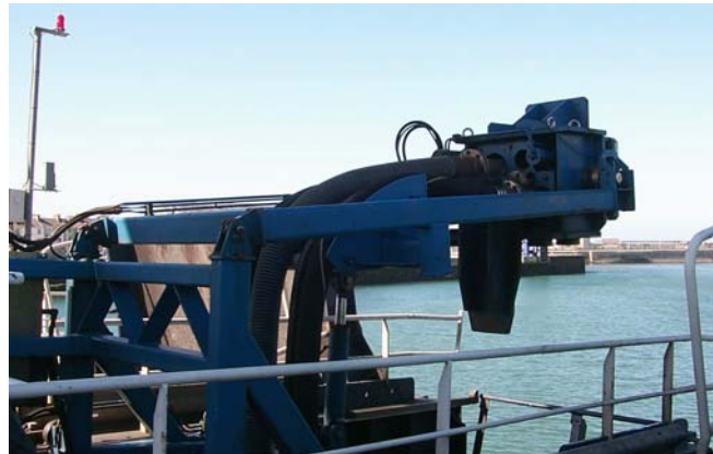
Figure 3.13 Manifold in Holyhead that provides HSS 1500 with fuel and fresh water and receives liquid disposals
