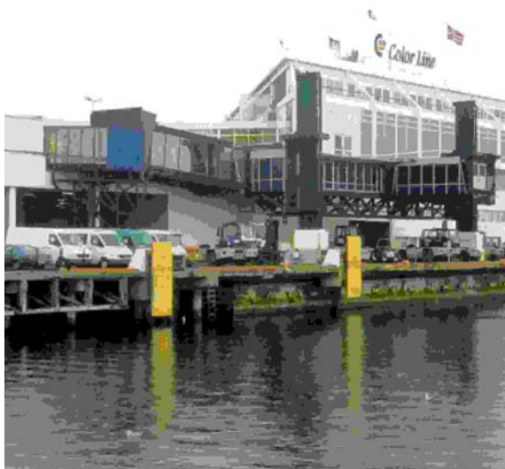
Figure 4.11. A flexible passenger gangway serving a rectangular area on the ship's side
