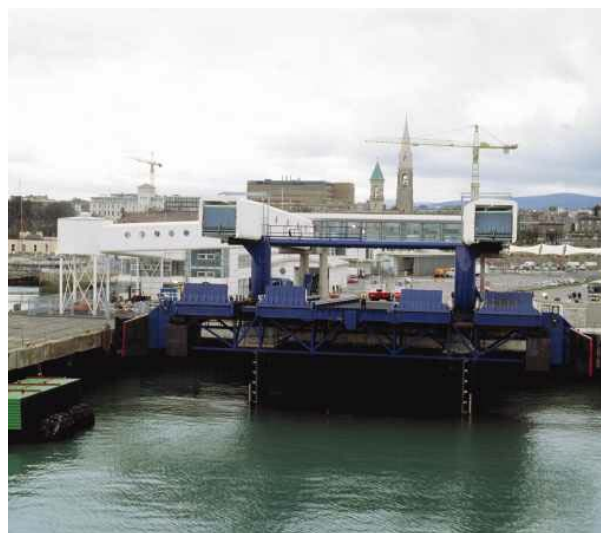
Figure 4.6. Linkspan for Stena Line Catamaran HSS 1500 in Dun Laoghaire, including passenger gangways
