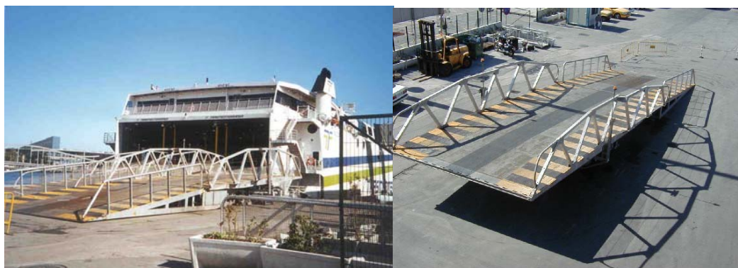
Figure 3.5 Ramp installed on land in the port of Barcelona for the Trasmediterranea Millennium
