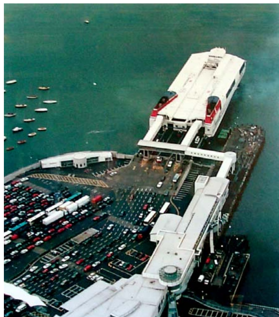
Figure 3.2 Stena HSS terminal in Dun Laoghaire, a purpose-built high efficiency port with high investment costs, and with a turn around time of around 20 minutes
