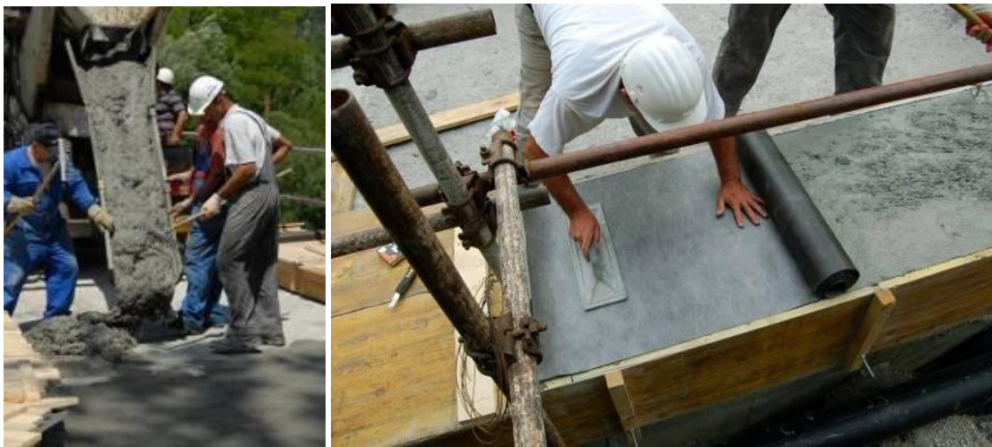
Figure 37 Processing of the materials on the site.
