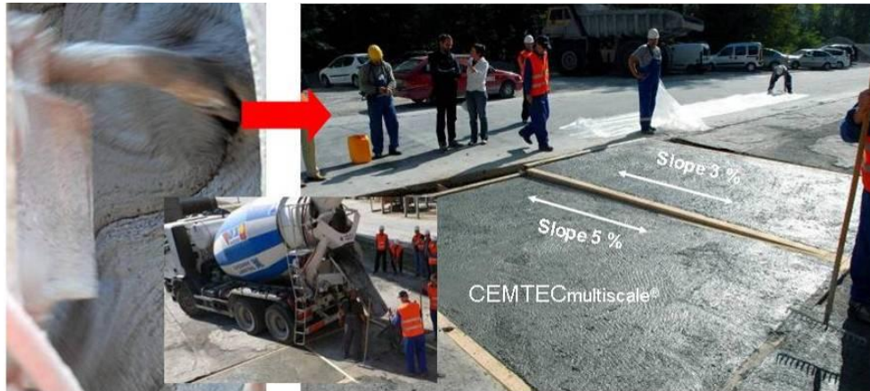
Figure 35 Full scale field trial, Salanit plant, Slovenia, October 2008
