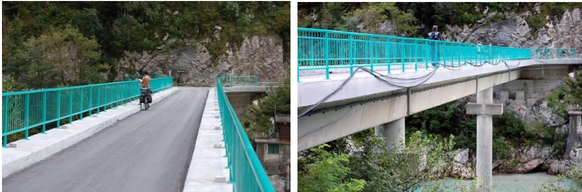
Figure 38 The bridge after the rehabilitation.
