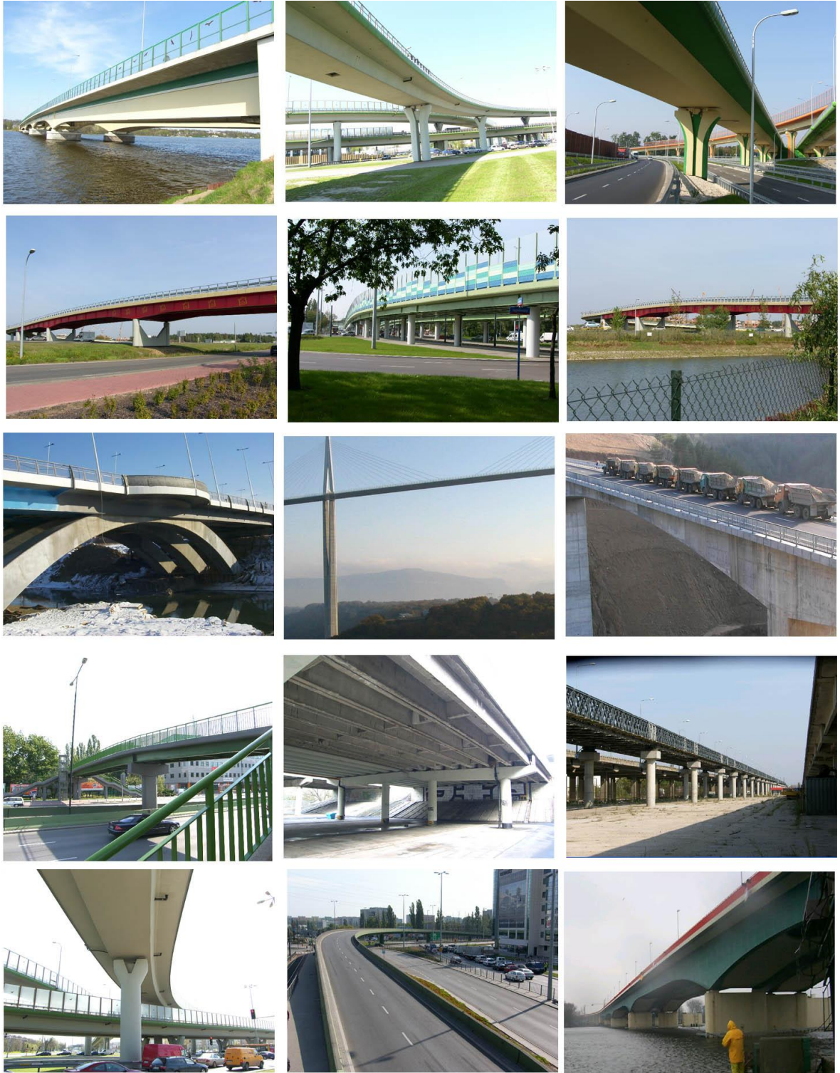
Figure 5 The example bridge photos
