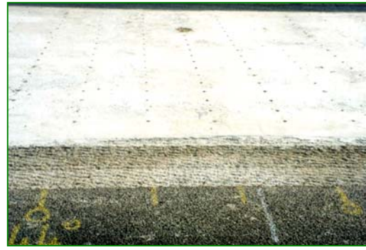
Figure 3 concrete slab of euphonic pavement
