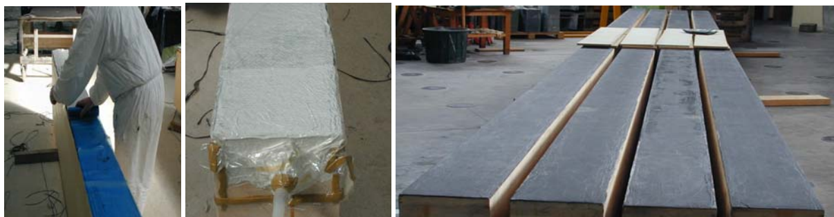
Figure 5 : Application of the CFRP reinforcement
