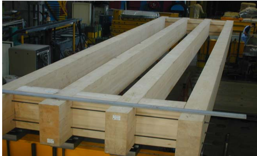
Figure 4 : Assembling the wooden beams
