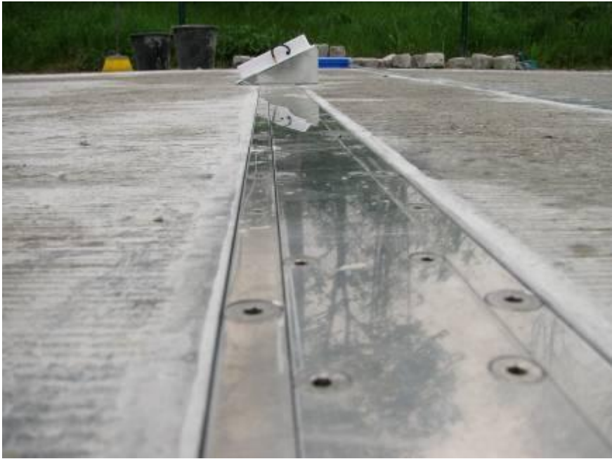
Figure 43: Installed prototype of new weigh-in-motion sensor.
