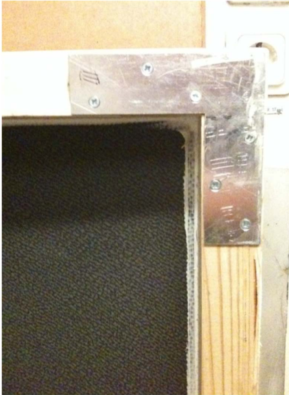
Figure 4 White mastic sealing the gap between the rubber mat and the wooden frame.
