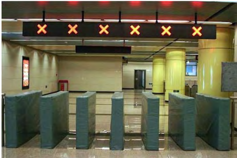
FIGURE 23 TELESCOPIC FLAP GATES
