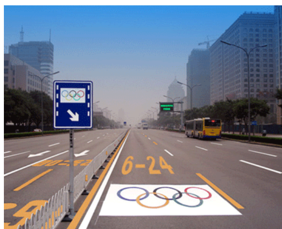
Figure 6.22 Example of Dedicated Lanes and signage on Beijing Olympic Route Network
