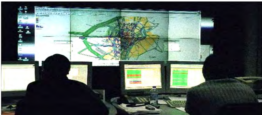
FIGURE 7 THE TRAFFIC OPERATIONS CENTRE
