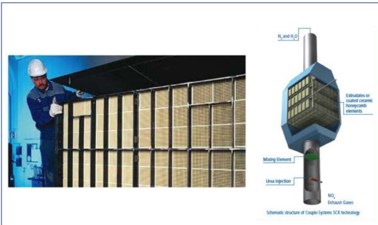
Figure 50: SCR ceramic elements during installation
