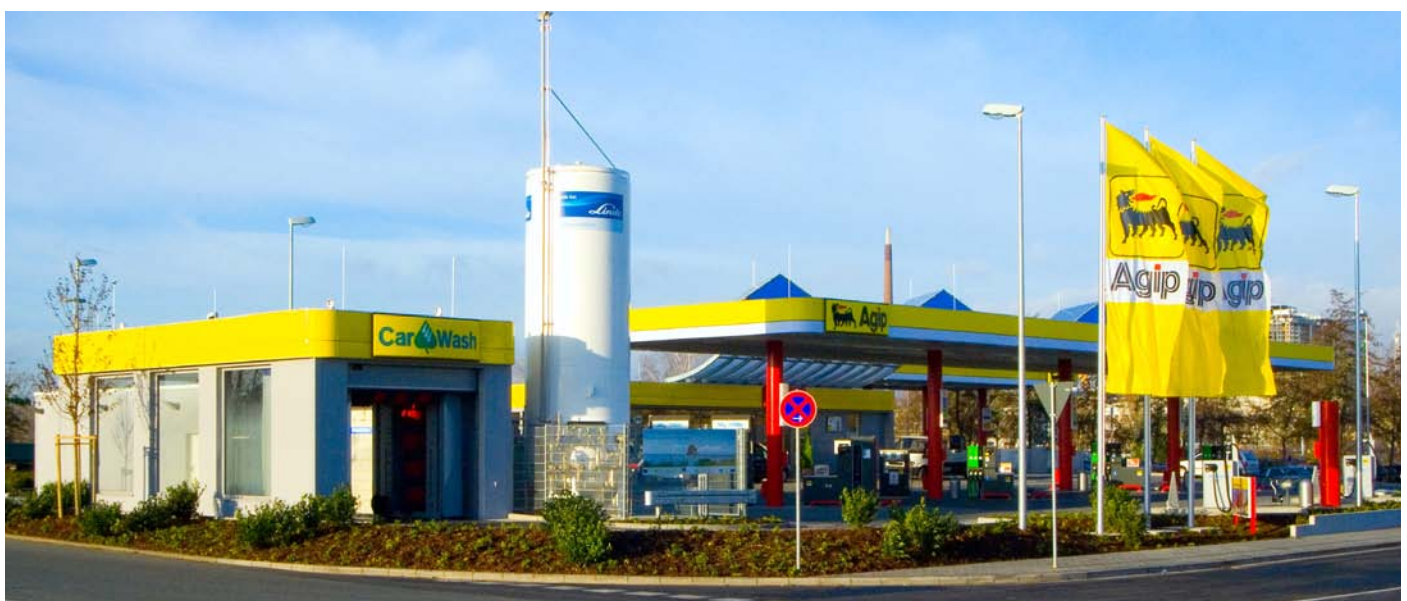
Figure 3: Agip service station in Frankfurt
