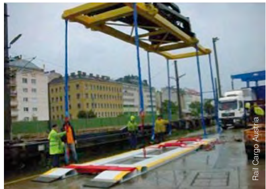
Figure 52: ISU loading platform and ropes connected to the crane spreader
