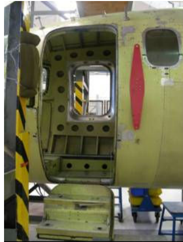
Figure 172: After repair the Pax Door repaired zone should be checked with a non destructive inspection (Liquid penetrant ) and reinstalled
