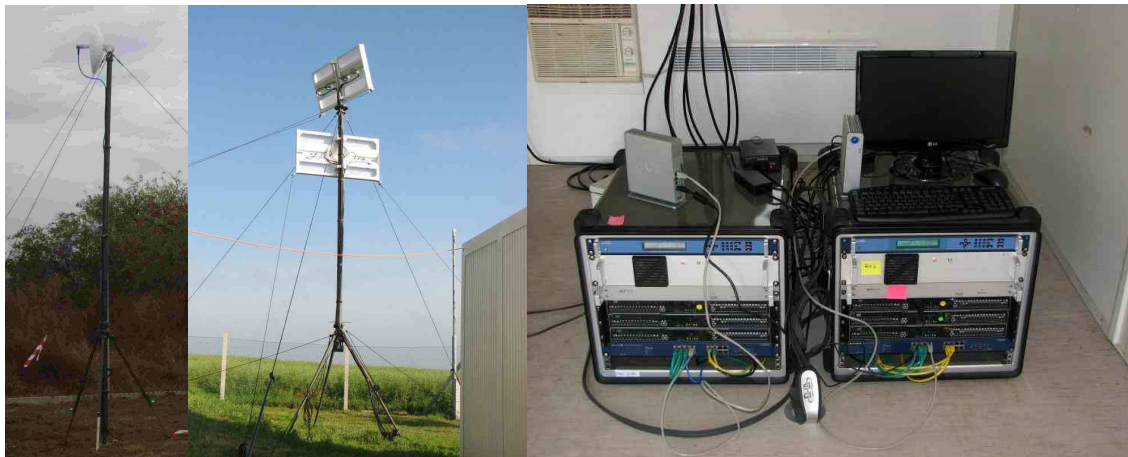
Figure 12. Borkovany installation, microwave data-link antenna, PCL antennas and receivers.
