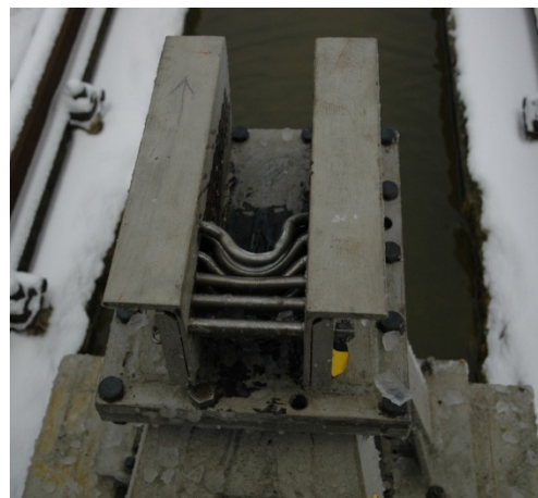
Structure of rotation device after the test
