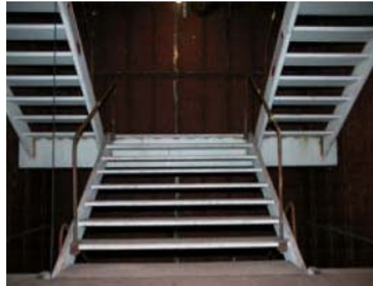
Figure 2.2-2 - I-Core™ stairs and staircase landings in cruise ships and deck houses.
