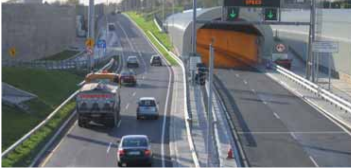
View of the South Bound Entrance of the Dublin Port Tunnel
