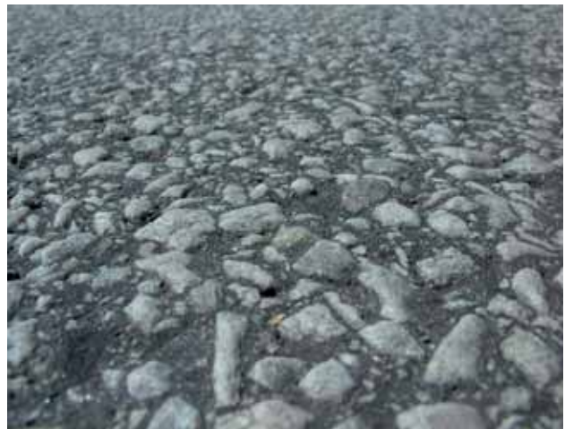
Thin layer surface from Ellenborgsvägen in Malmo Photo: Danish Road Institute
