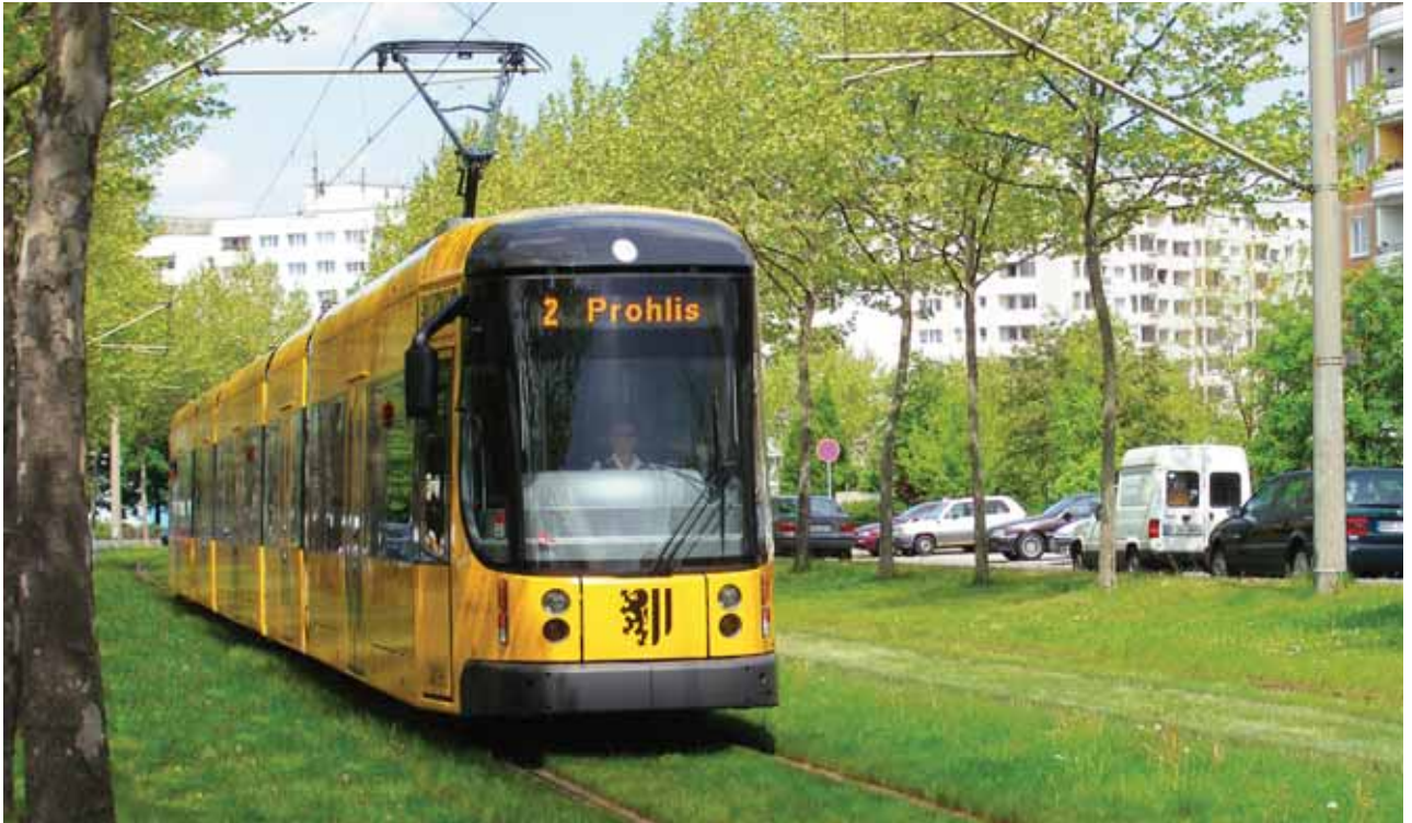
Tram on lawn tracks in Dresden, Germany
