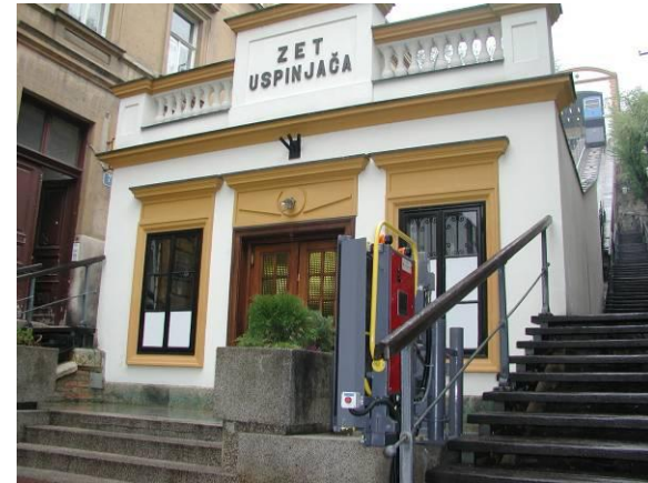
Adjusting old building, Zagreb
