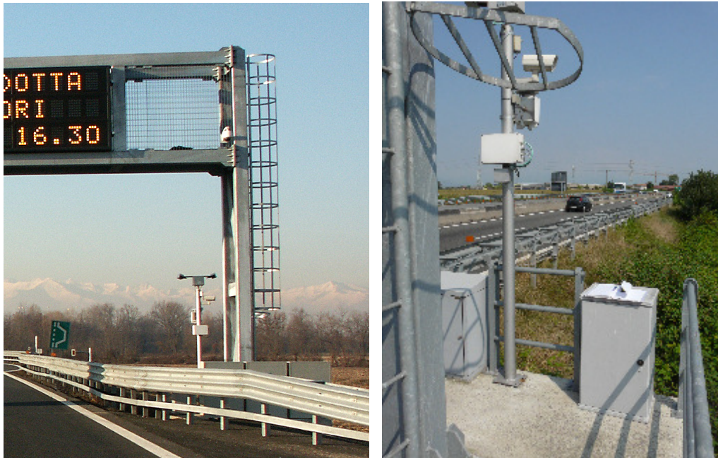
Figure 28: The Turin- Airport freeway
