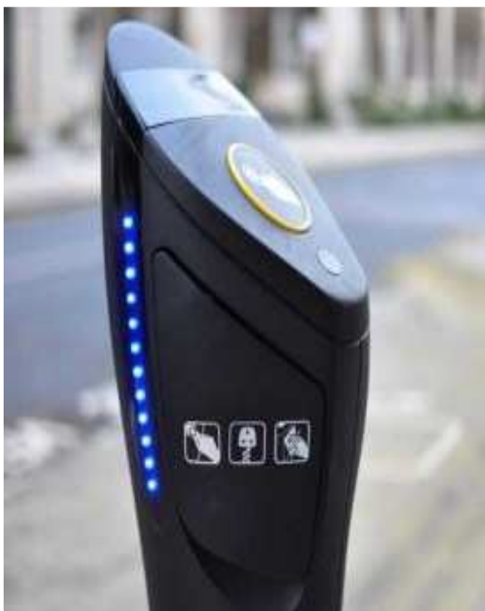
Figure 24 – An on-street POD Point. Note the protective door and the RFID reader (yellow circle) [16]
