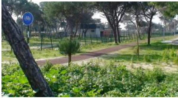
A finished part of the cycleway
