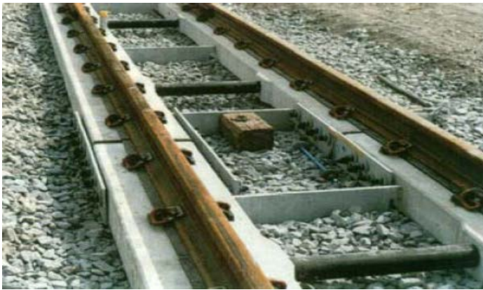
fig. 8: a typical laddertrack setup with ballast
