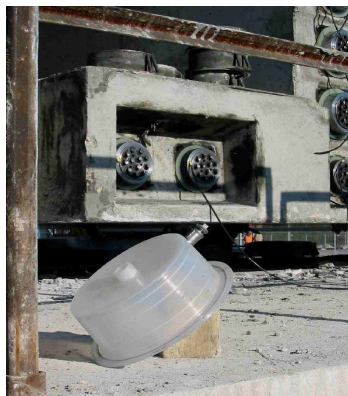
Figure 16: Piacenza viaduct anchorage and transparent stocking area [23] Figure 17: Piacenza viaduct full span precast deck in anchorage [18].
