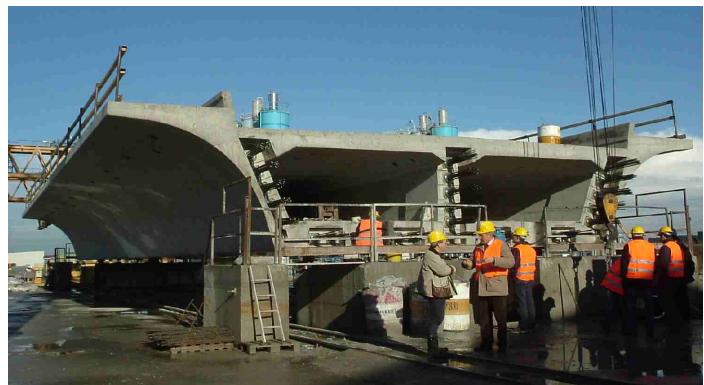
Figure 16: Piacenza viaduct anchorage and transparent stocking area [23] Figure 17: Piacenza viaduct full span precast deck in anchorage [18].
