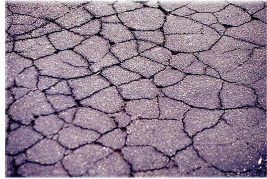
FIGURE 11: Fatigue cracking.
