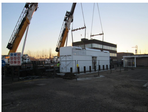
Figure 1: Installation of the HRI at the Solvay plant in Antwerp.
