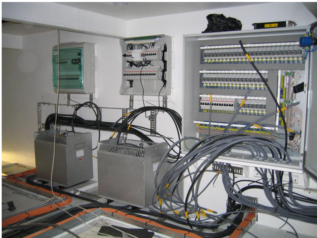
Illustration: More pictures from the installation process.
