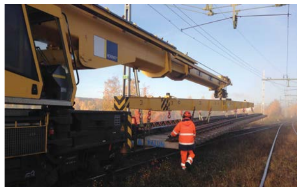
Figure 2 – S&C panel transported by a KIROV crane in Falun in Sweden
