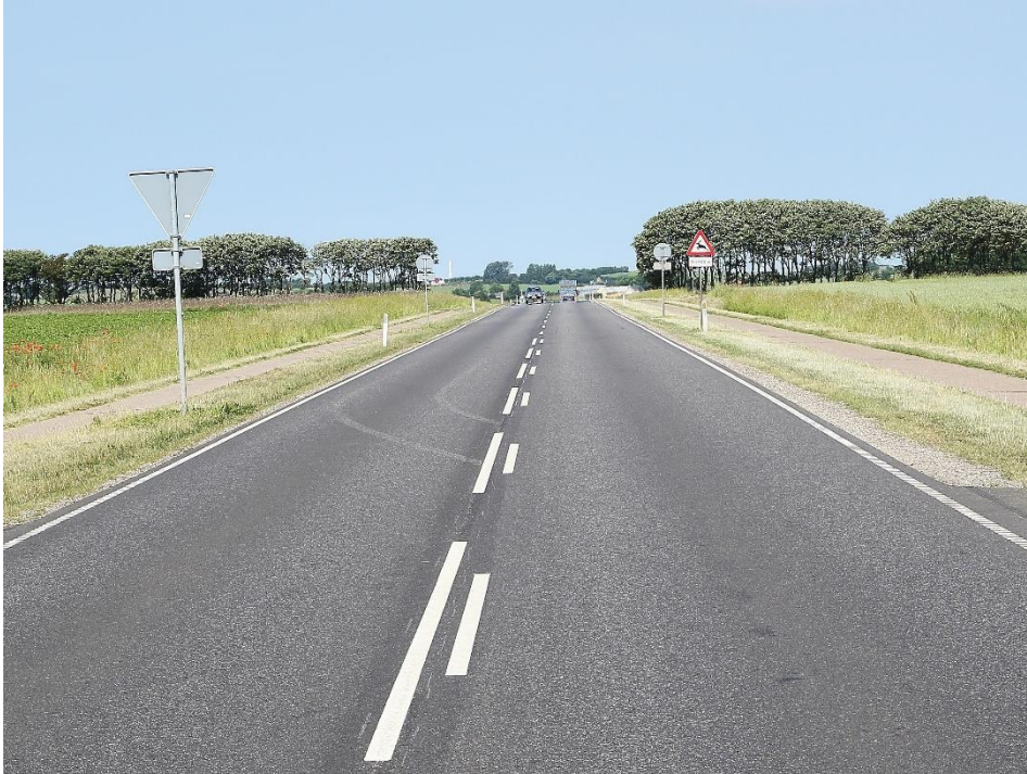
Figure 5: The road used for the Danish test site. Photo: Trond Cato Johansen, Ramböll.
