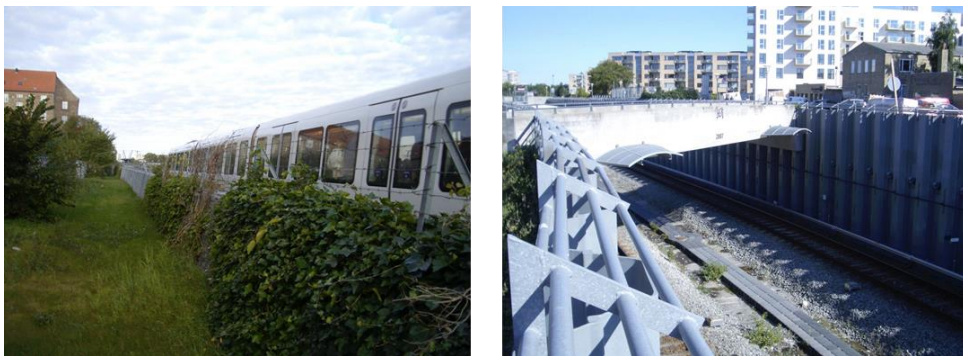
Figure 6: Example of fencing and bridge protection
